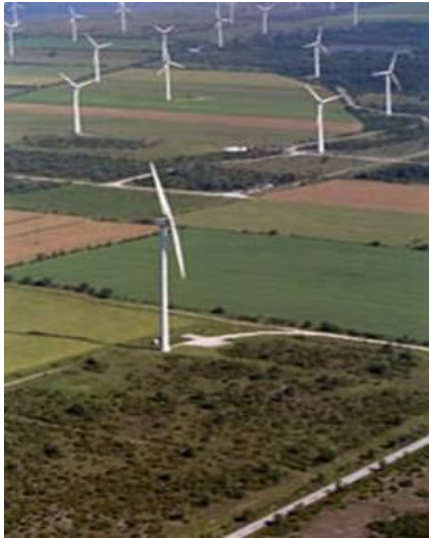
20MW Wind Farm
