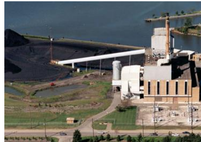
22MW Biomass Conversion JDY - U5
