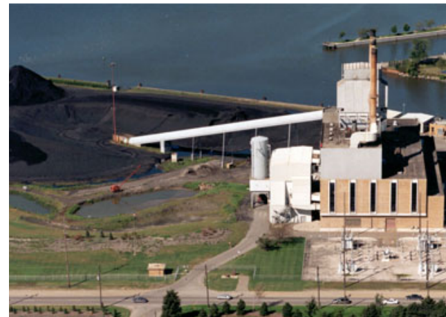
22MW Biomass Conversion JDY - U5
