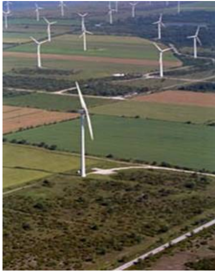
20MW Wind Farm
