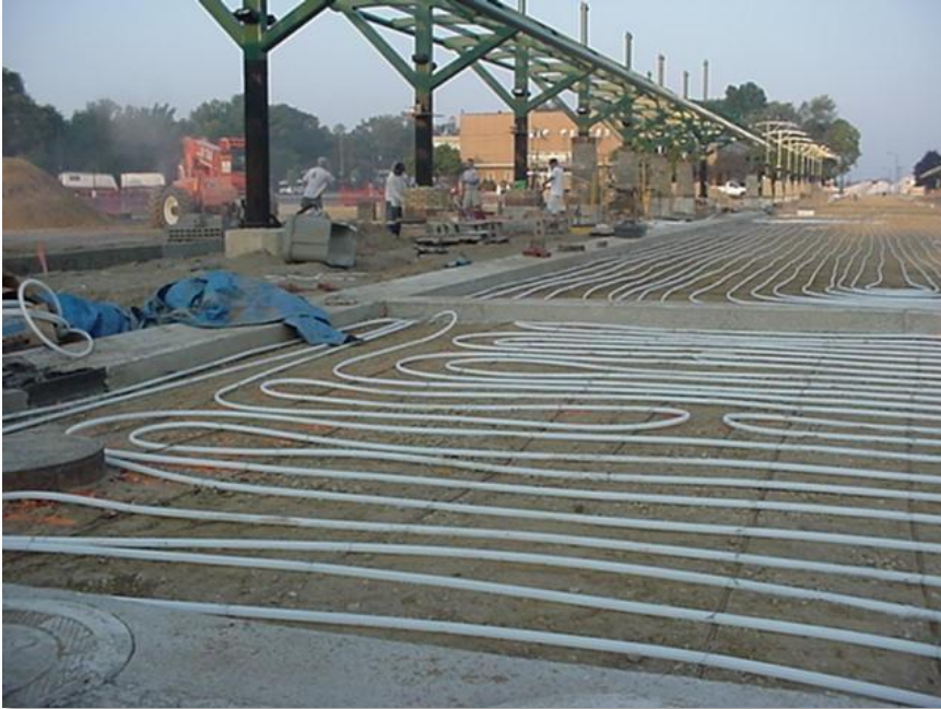
Installation of Snowmelt on 8th Street at Marketplace
